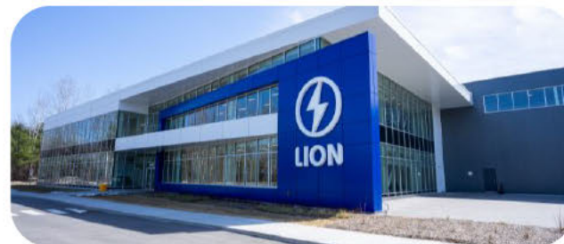
BATTERY PLANT IN MIRABEL, QC
