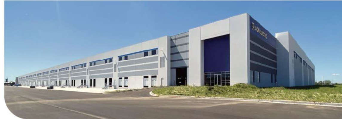
MANUFACTURING FACILITY IN JOLIET, IL
